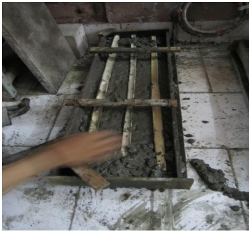
Figure 10 Placing of bamboo in singly reinforced slab panel
