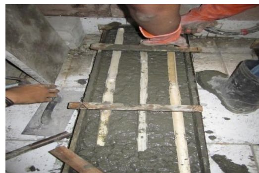
Figure 13 Casting of concrete slab panel with bamboo reinforcement
