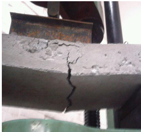
Figure 16 Development of the crack in singly reinforced slab panel
