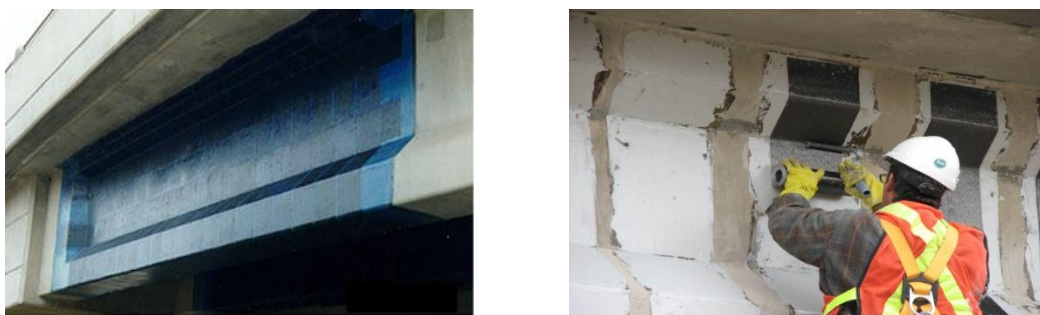
Figure-1. Shear strengthening of Reinforced concrete using CFRP laminate.
